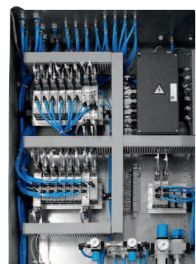
Magnetventilschrank Zone 1/21
